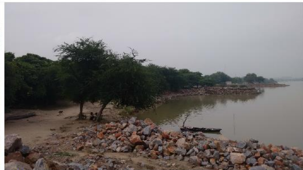
View of ongoing shoreline construction activities at site
