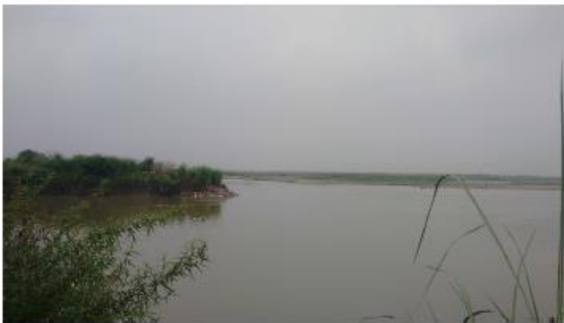
View of river and shore protection at site
